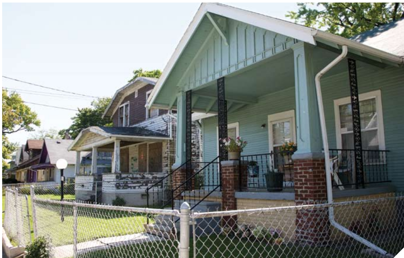
Flint’s shrinking population and declining economy have resulted in abandoned housing next to well-maintained homes.
