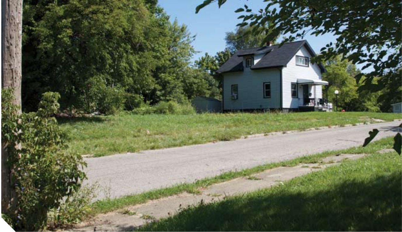
▼ In some Flint neighborhoods, occupied housing is now surrounded by empty lots because of demolition of dilapidated buildings by the Genesee Land Bank.
