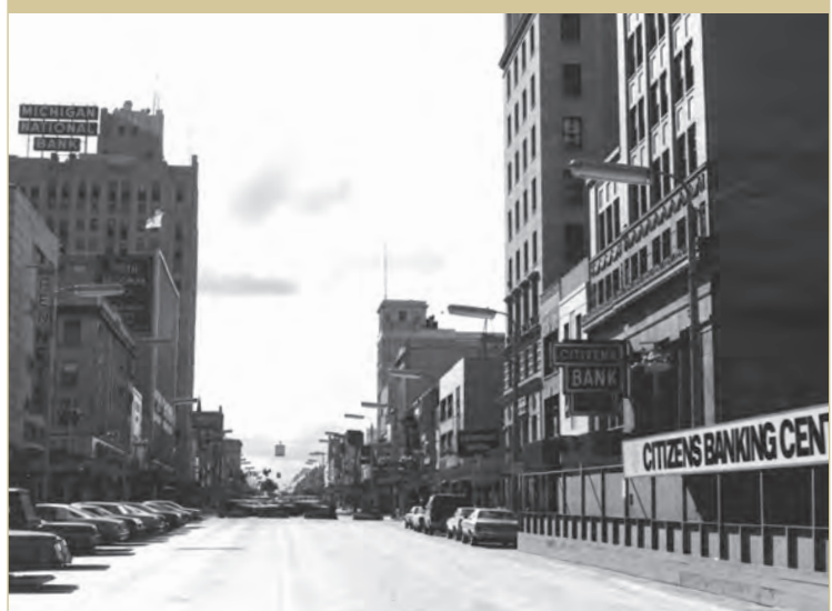
New construction in the central city - 1978.
