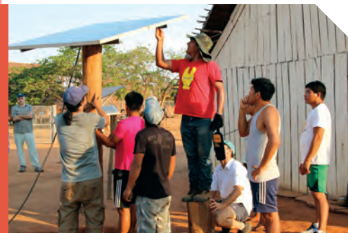
Installing solar panels in Pyulaga Village, Brazil – 2016.
